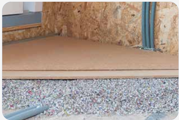
THERMOFLOC insulation pellets as cellulose granules resistant to compression
